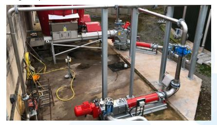
Marches Biogas were asked by Austrey Farm AD to install a Vogelsang PreMix feed system as a replacement to the existing Vogelsang QuickMix feed system, in order to reduce running & maintenance costs, and increase reliability of larger feed volumes.
